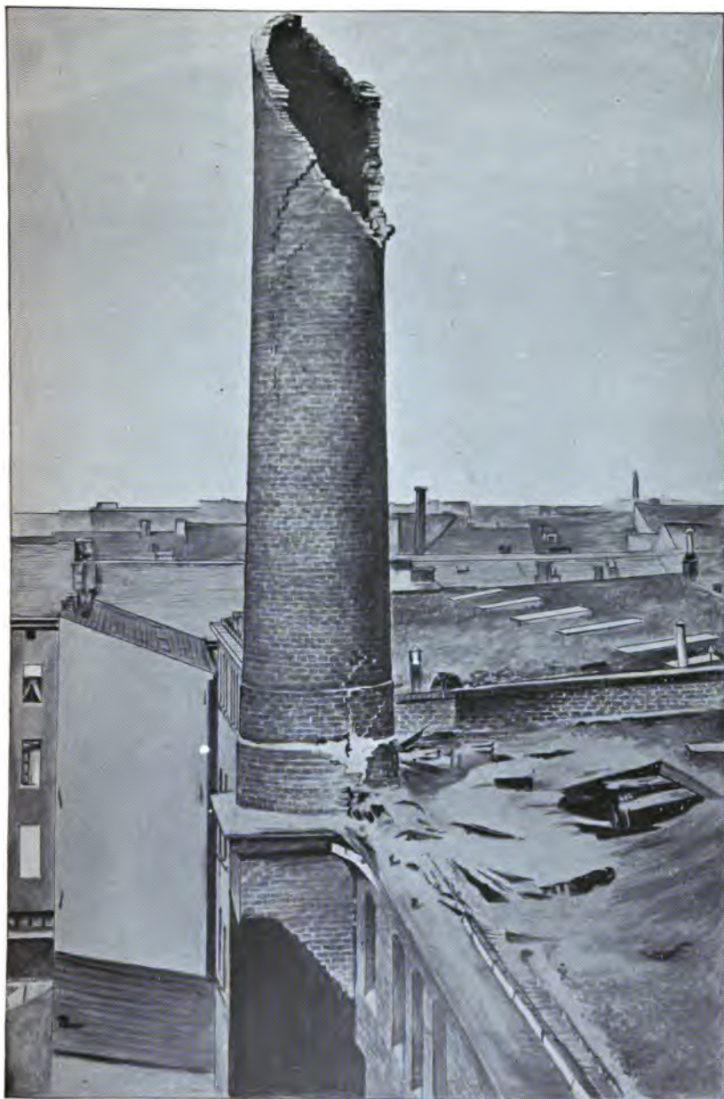
Fig. 5. Chimney, struck July 29, 1890. From Elec. Zeits. , Grebel.
